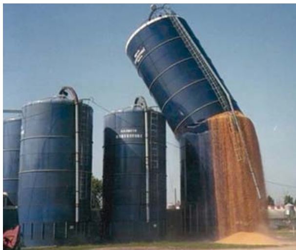
Rysunek 1.5. Awaria silosu z kukurydzą ( http://farminjuryresource.com/2018/04/18/grain-silo-accident-kills-father-and-son/ )
